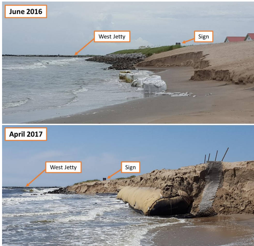
Figure 5. Field pictures show the increase in erosion on western end of Grand Isle. Pictures taken from west walkover looking toward the west jetty in June 2016 (top) and April (2017).
