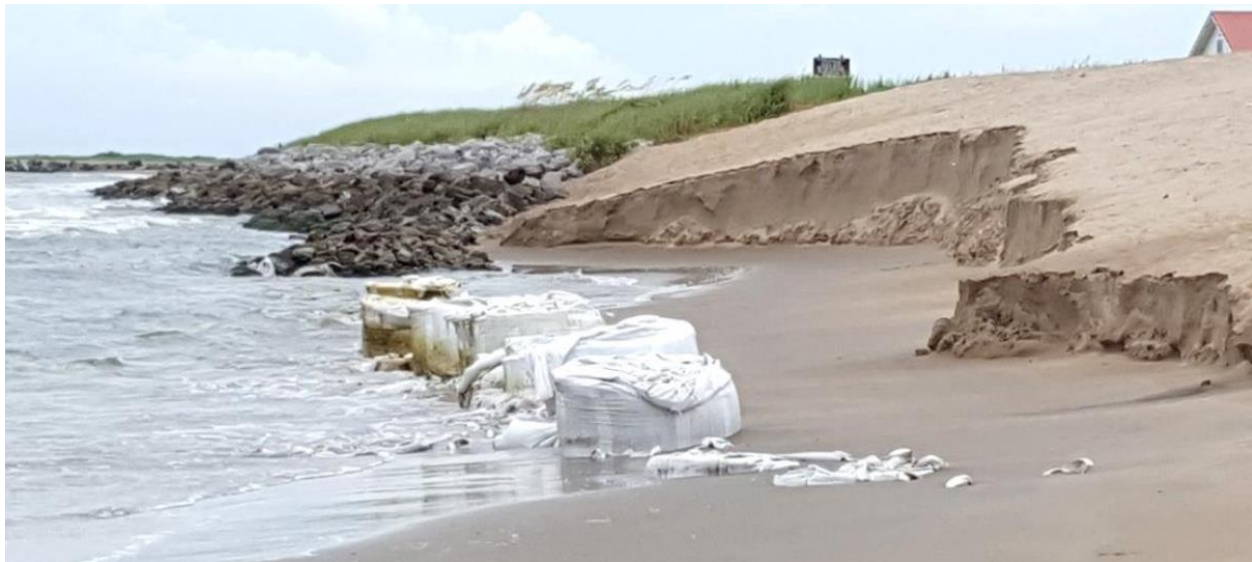
Figure 20. Northern end of rock revetment, existing scarp is indicative of severe erosion. Picture taken on July 2016 looking towards the southwest.
